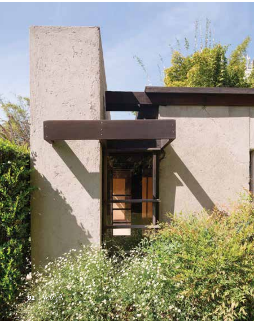
Below: This detail of the Kings Road house shows a redwood element that acts as a sun-shading device. Opposite page: Although outdoor fireplaces and fire pits are now common features of homes in Los Angeles, Schindler was among the first architects to incorporate them as details. Most of the large concrete walls were cast in place. Photos courtesy of the MAK Center for Art and Architecture
